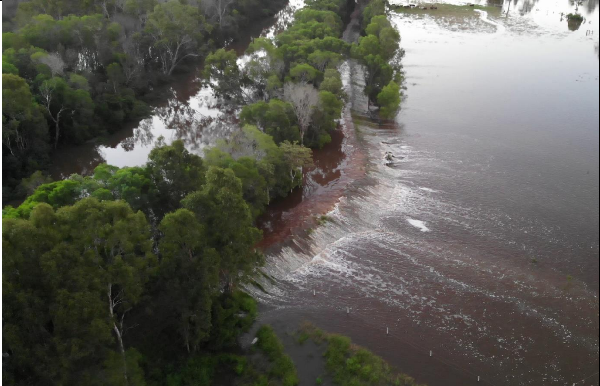
Image 2 - Looking south-east after major breach in levee has occurred - 2021.
