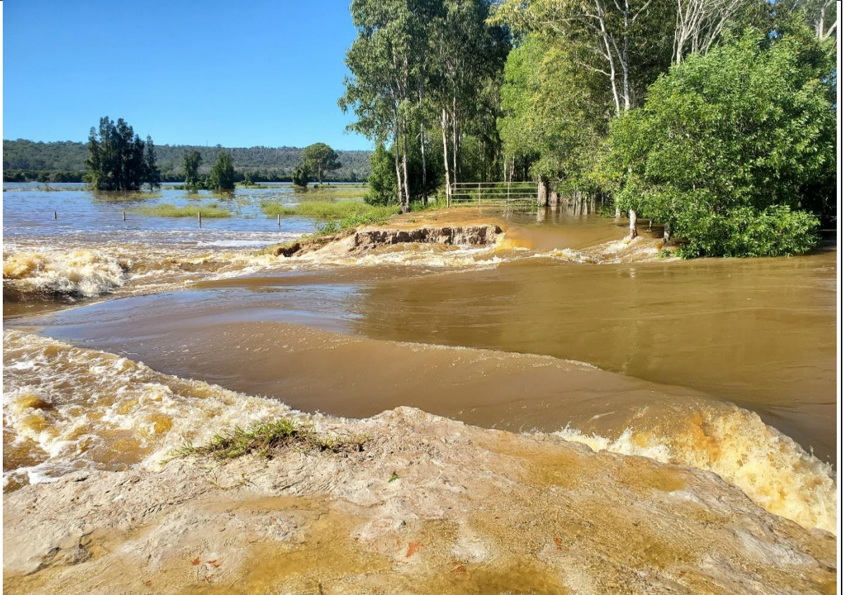
Image 2 - Looking south-east after major breach in levee has occurred - 2021.
